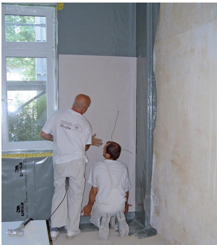
**8** Mounting of a second plaster board as ground for painting, wallpapering or tiling.
