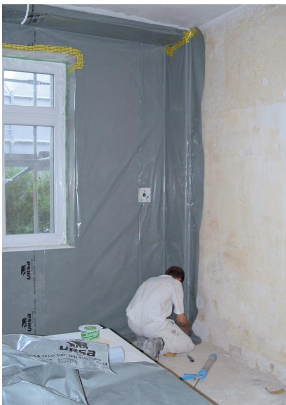
**7** Vapor retarders have to be mounted uninterruptedly over the insulating wedges in integrated inner walls and ceilings, as well as in reveals.
