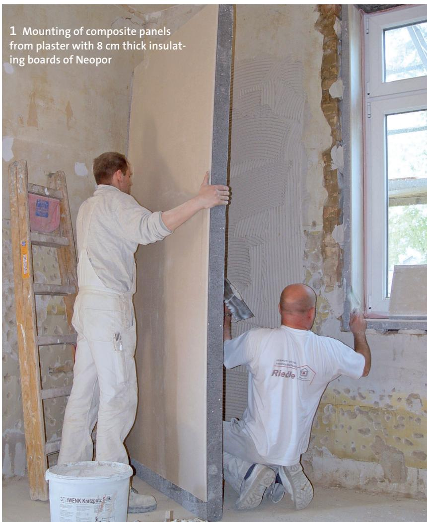
1 Mounting of composite panels from plaster with 8 cm thick insulating boards of Neopor
